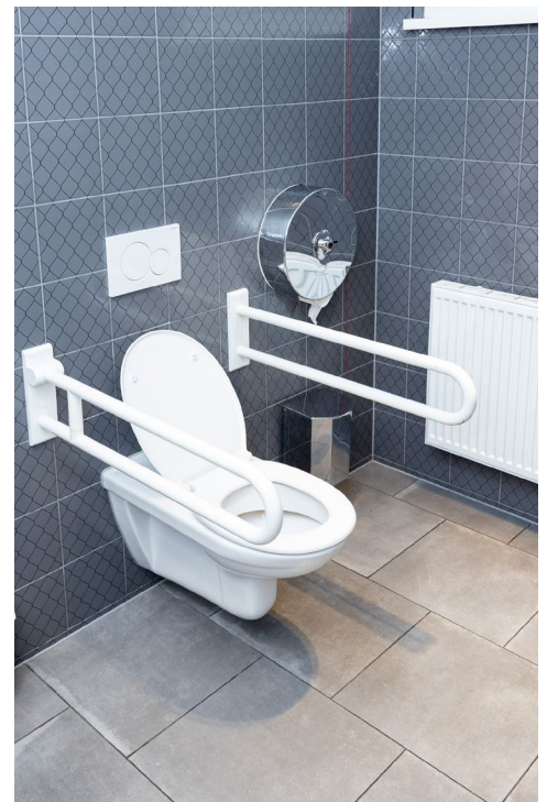
General accessible WC
