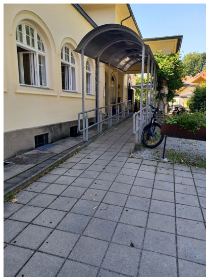
Access and ramp
