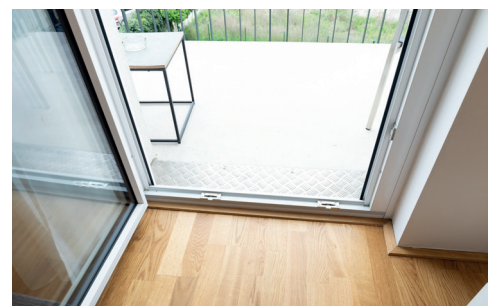
Access to balcony
